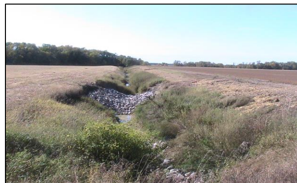
Drop Structure in Laterals of JD 29
