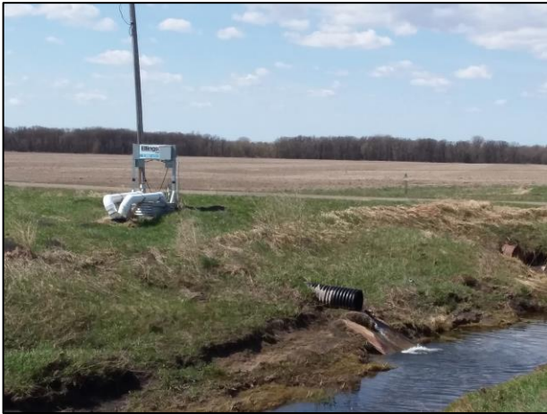
Example of a well-designed tile sump pump and pipe infrastructure emptying into Judicial Ditch 20 Branch A SW4 section 19 Vega Township
