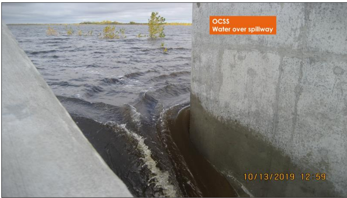
The Off-Chanel Storage Site located in section 15 & 16 of Comstock Twp was also at full capacity in October. The site diverts high water from the Snake River that is ultimately diverted around the City of Warren.
