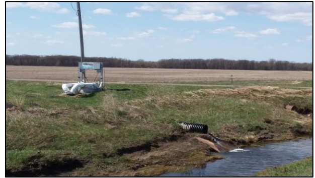
Example of a well-designed tile sump pump and pipe infrastructure emptying into Judicial Ditch 20 Branch A SW4 section 19 Vega Township
