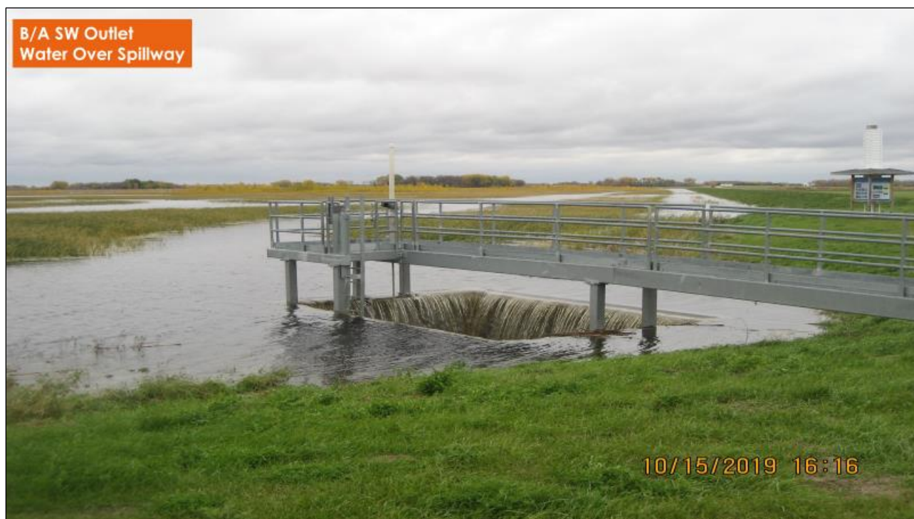
The southwest outlet structure of Brandt/Angus Impoundment site reached maximum gated storage level in October. Water remained in the site until late November.
