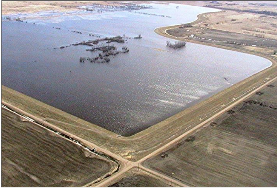
Figure 1 Agassiz Valley aerial photo looking southeast, the outlet structure is located at the bottom of the photo. JD #25-1 is the ditch that Agassiz outlets into, which flows to the Snake River.
