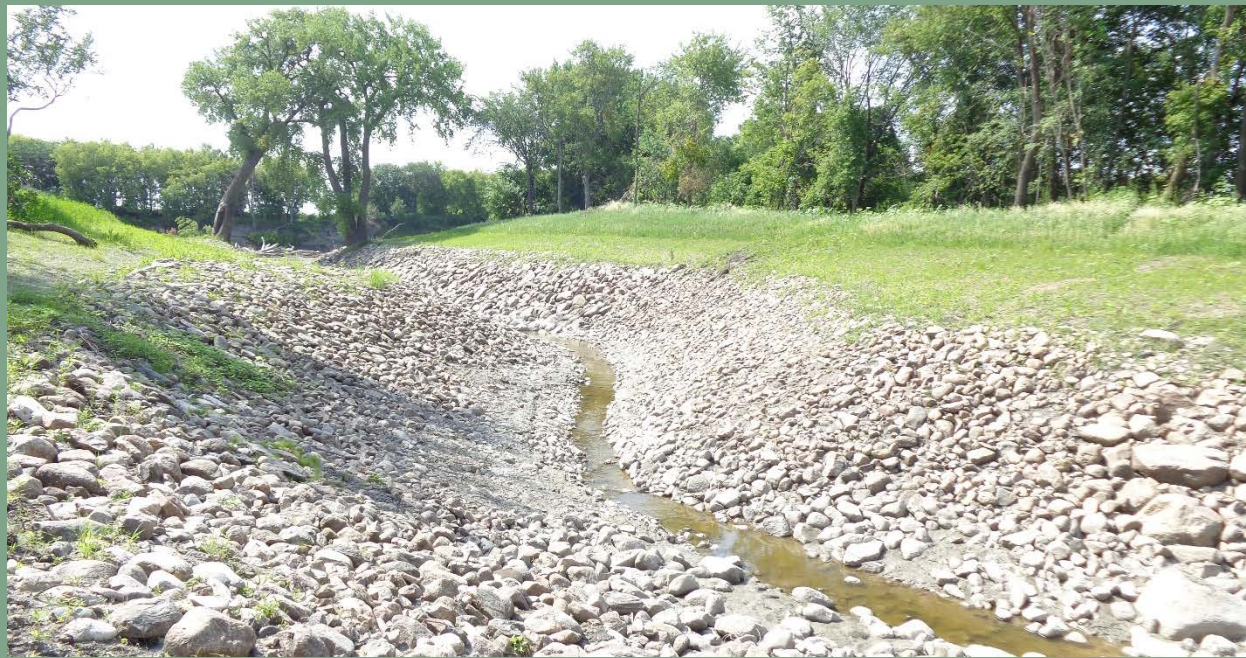
Grand Marais stream restoration, 2014
