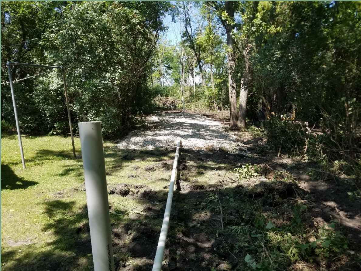
Subsurface Sewage Treatment System (SSTS) at grade construction in Polk County
