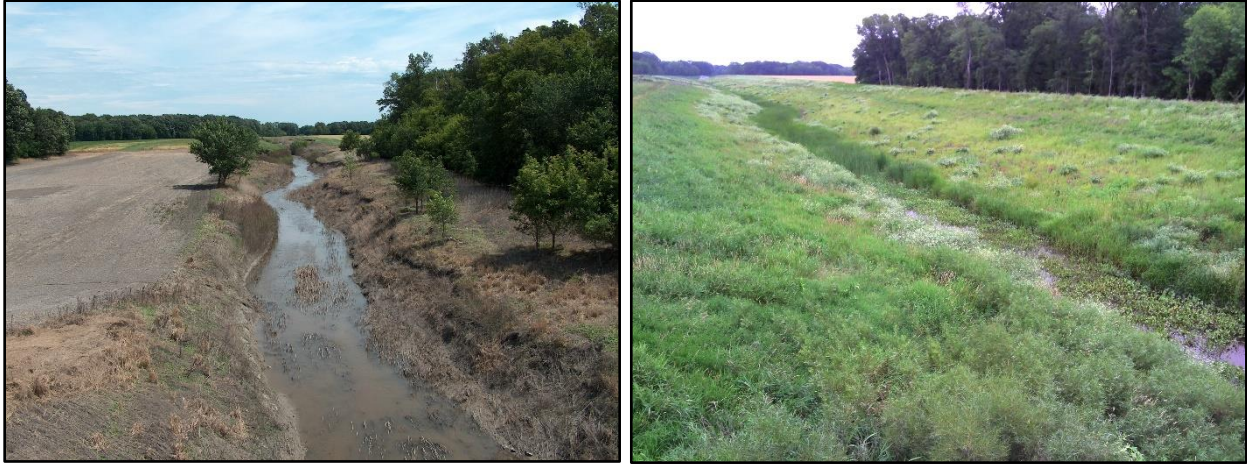
Figure 1-4. Grand Marais Creek Cutoff Channel, looking upstream of County Road 64 before (left 2007) and after (right 2016) the Grand Marais Creek Cutoff Channel Stabilization Project.
