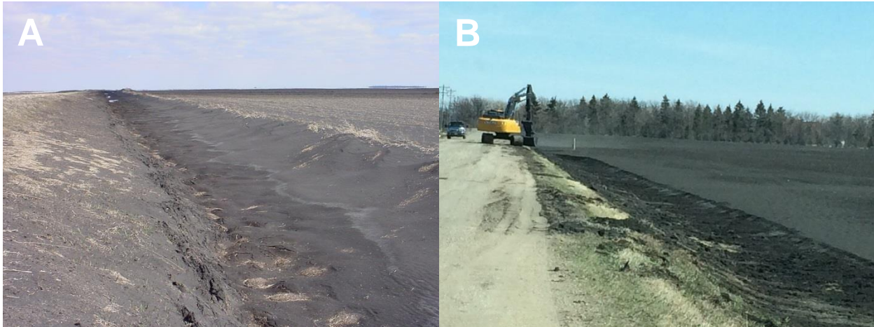
Figure C1: Photos illustrating (a) edge-of field wind erosion following a high wind event, and (b) ditch maintenance to remove eroded sediment.
