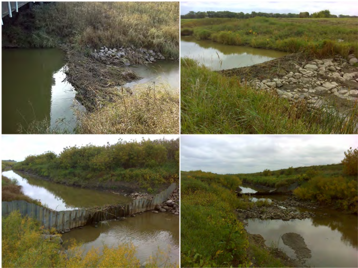
Figure 25. Photos of connectivity barriers along AUID 520, including a beaver dam at the State Highway 220 crossing on November 5, 2013 (upper left); a beaver dam immediately downstream of the confluence with CD 7 on September 24, 2014 (upper right); and grade control structures immediately upstream of the confluence with the Red River of the North on September 24, 2014 (lower left and lower right).
