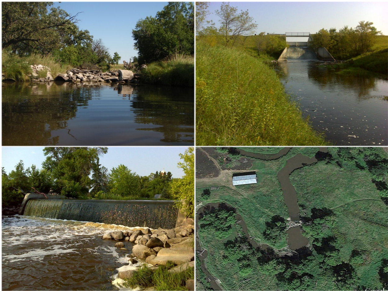
Figure 8. Photos of connectivity barriers along AUID 503, including the remnants of a private stream crossing at Station 08RD031 on September 3, 2008 (upper left); the Florian Dam on September 2, 2015 (upper right); the Stephen Dam on July 30, 2014 (lower left); and the remnants of a private stream crossing downstream of the 330 th Ave. NW crossing on September 1, 2013, courtesy of Google Earth (lower right).
