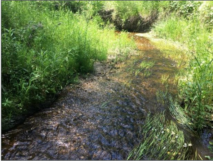
Figure 11-8: Existing Outlet Channel
