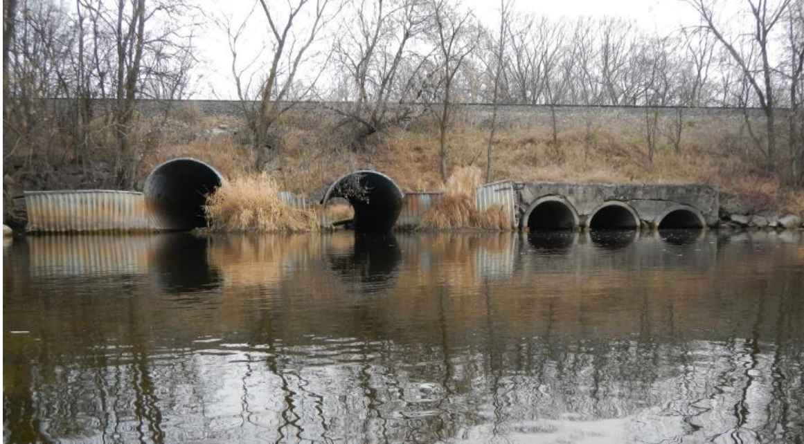
Figure 7-2: Existing Railroad Structures at Newfolden
