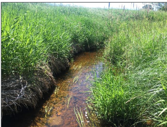
Figure 6-8. Erosion of Existing Channel
