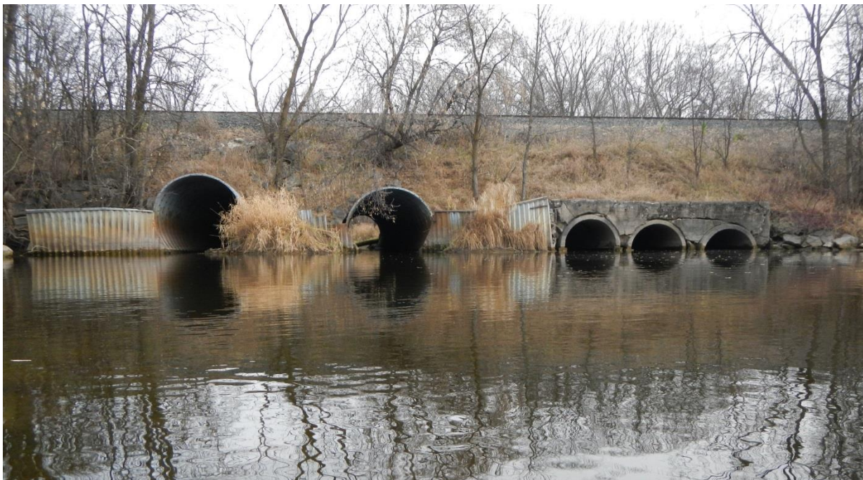
Figure 4-3. Existing Railroad Structures at Newfolden
