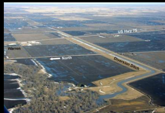
DIVERSION CHANNEL (RICHARD P. NELSON FLOODWAY)
