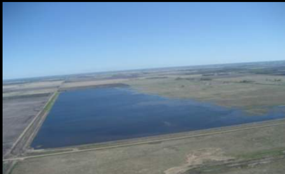
RETENTION SITE (BRANDT ANGUS IMPOUNDMENT)
