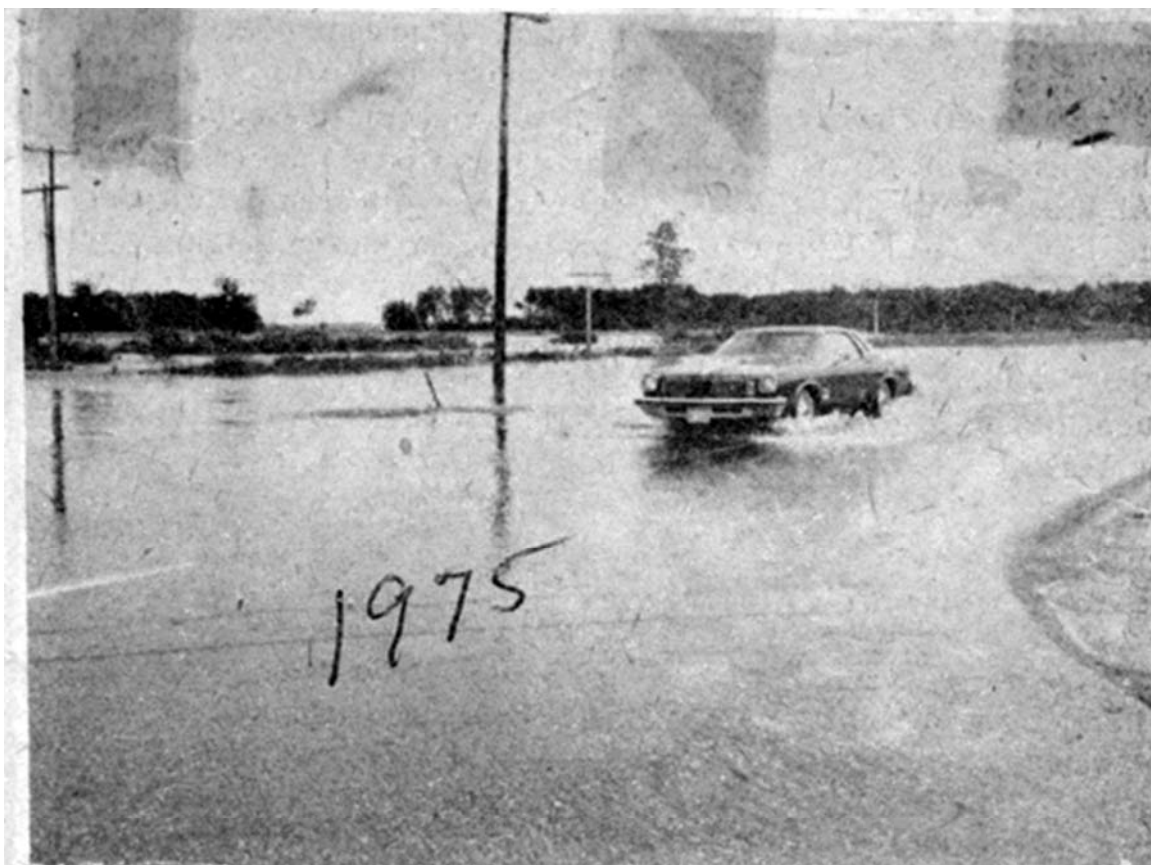
Traffic was slowed Wednesday on highway 59 four miles south of Newfolden as water was flowing over county road seven as well as highway 59. The Soo Line tracks near this intersection were under water as gravel under the rails washed away.
