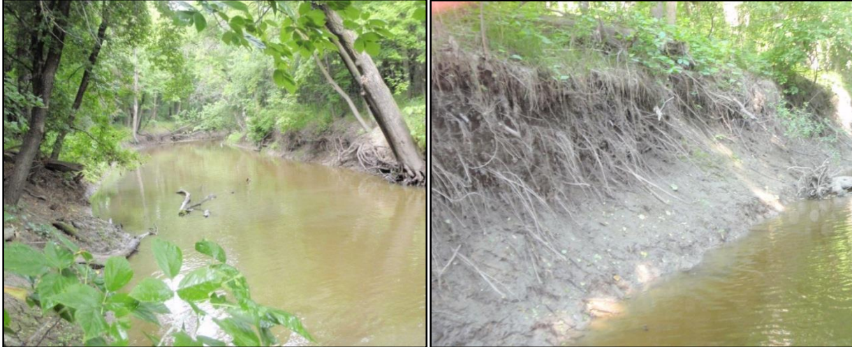
Figure 22. Sloughing trees and bank erosion at 94RD511.
