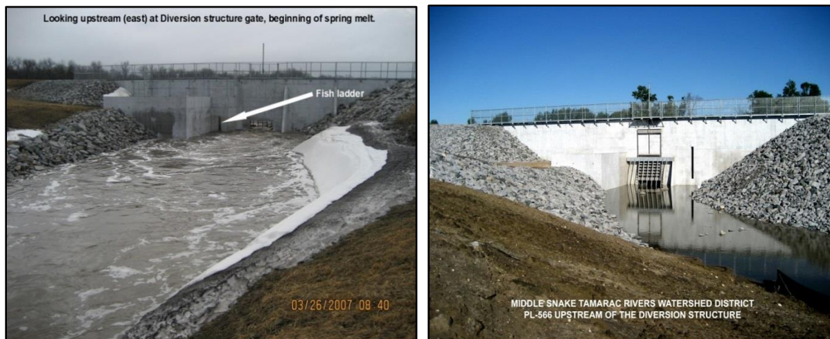
Figure 18. Dam on the Snake River upstream of Warren during high (left) and low flows (right) and the location of the fish ladder (photos courtesy of MSTWD 2009).
