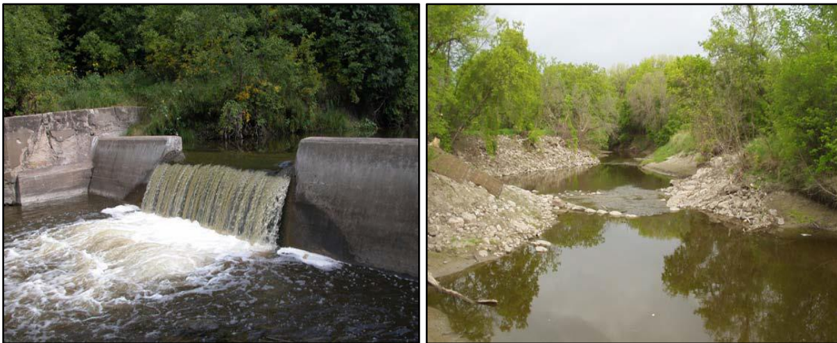
Figure 29. Before and after pictures of the Middle River Dam in Argyle, Minnesota (Photos courtesy of MNDNR).
