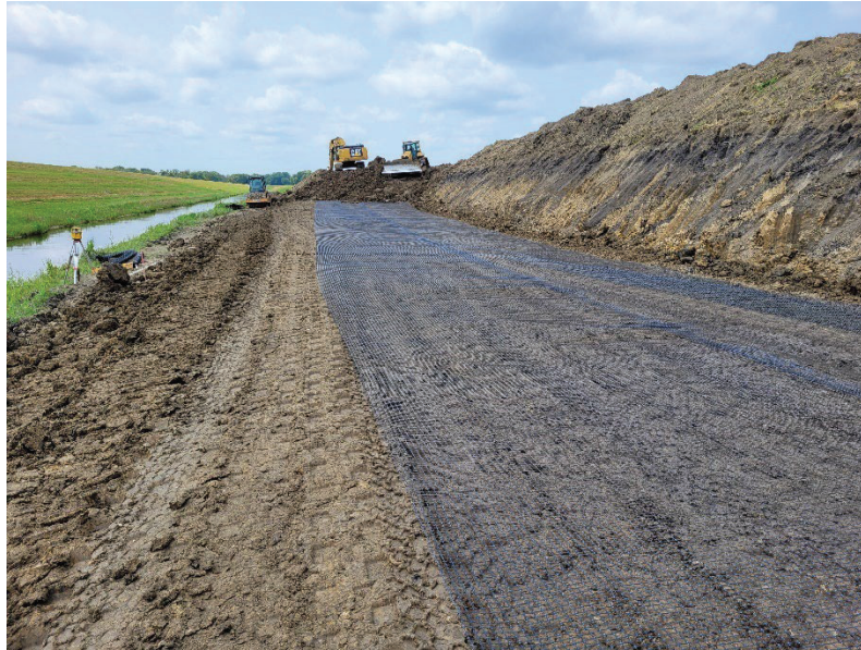
Layers of Geogrid being installed in the Road Slope of JD 75
