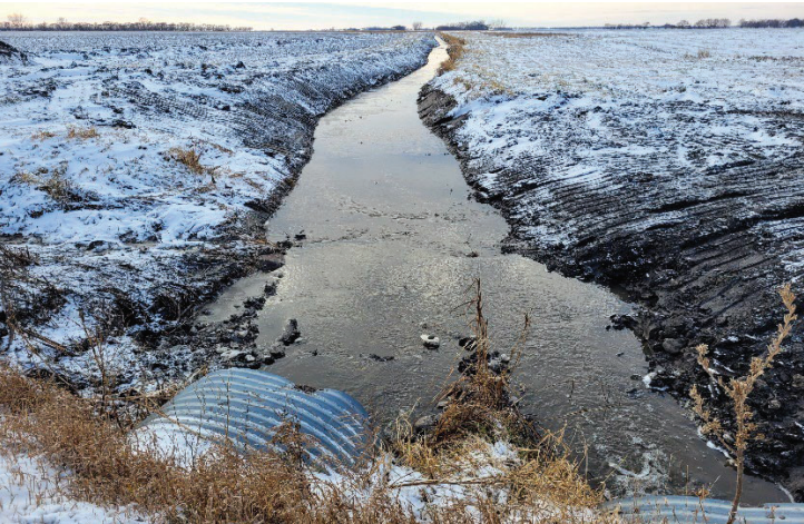
Looking East at the Brandt Angus Coulee following sediment removal in Section 28 Angus Township. Most of the Coulee downstream of the Impoundment had not seen any maintenance since planning for the Project had begun in the mid-2000s.
