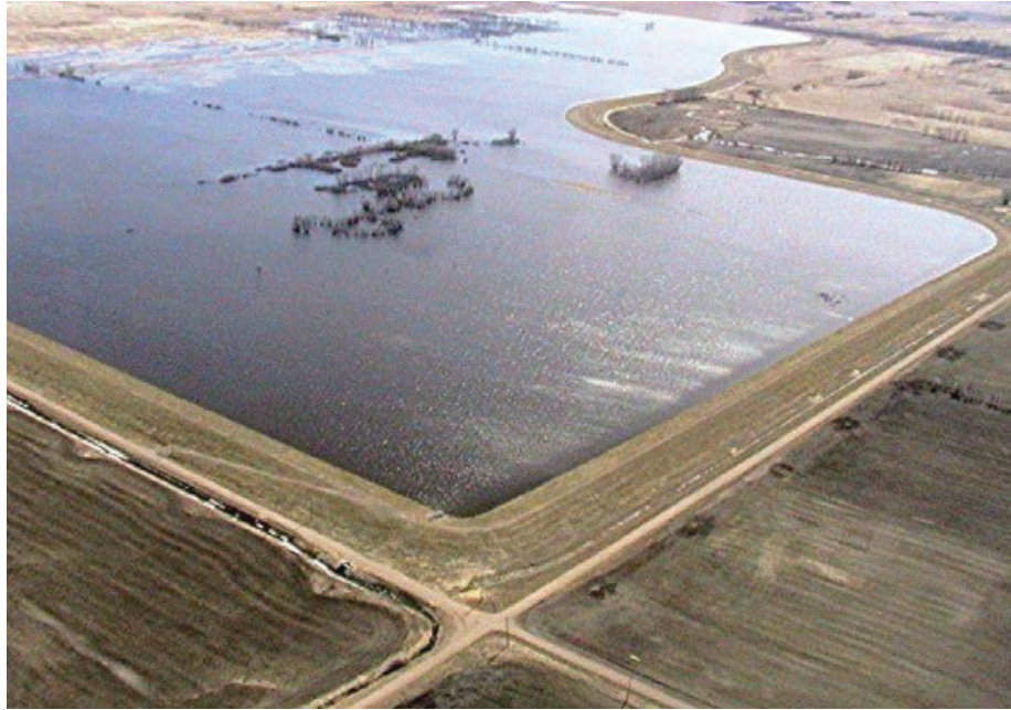
Figure 1- Agassiz Valley aerial photo looking southeast. The outlet structure is located at the bottom of the photo. JD #25-1 is the ditch that Agassiz outlets into, which flows to the Snake River.
