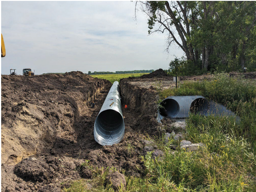
Looking NE at BAC North Inlet. A third 48" culvert was installed under 260 th Ave. Upstream landowners had expressed concerns to the District with ponding that was occurring on their property from water that could not enter the project quick enough.
