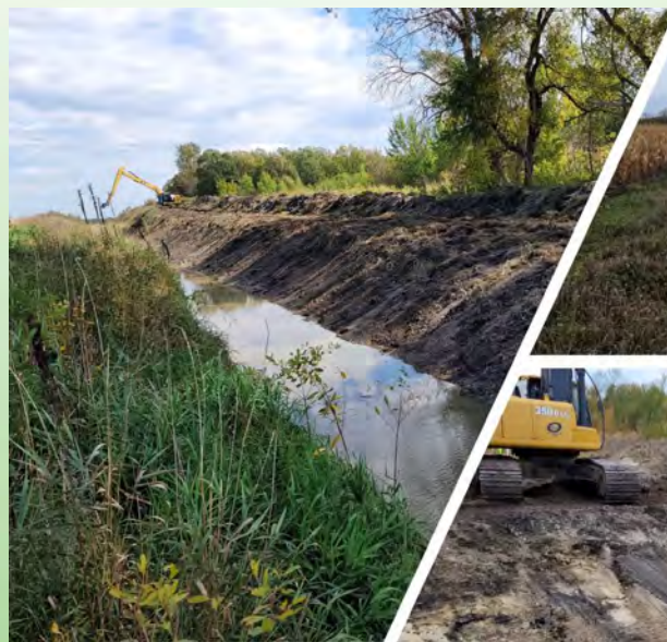
Sediment Removal on Judicial Ditch 14
